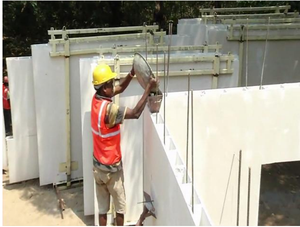
FILLING CONCRETE BETWEEN PANEL
