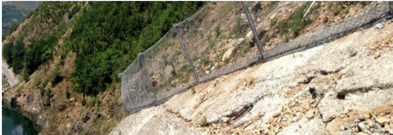
Figure 3. Protective structure against landslides
