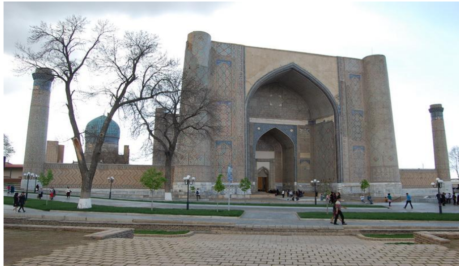
Figure 6 Renovated front view of Bibi Khanum Mosque
