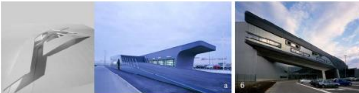
FIGURE 1. CREATIVE WORKSHOP "ZAHA HADID ARCHITECTS" (ZHA): A) BMW SHOWROOM 2003-2006, B) BMW CENTRE 2001-2005.
