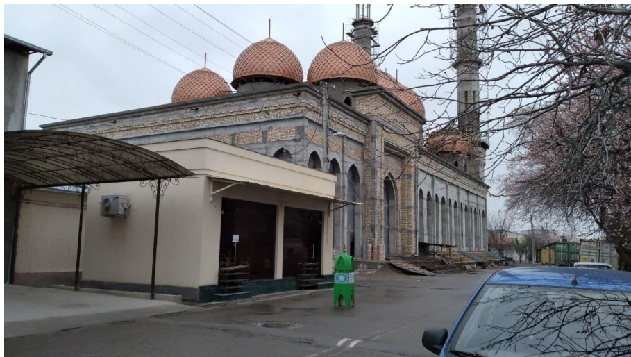
Figure 5 This is the building of the Rakaat Mosque under construction today.
