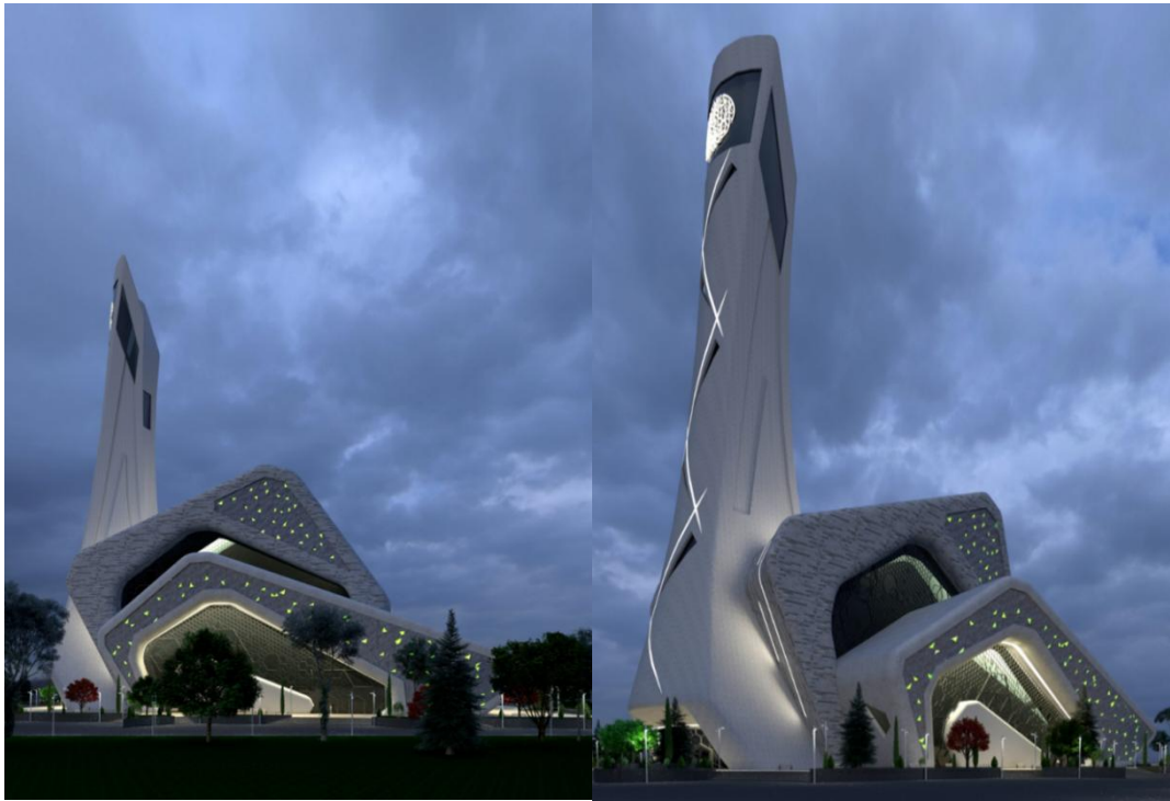
Figure 6 General view of the building.
