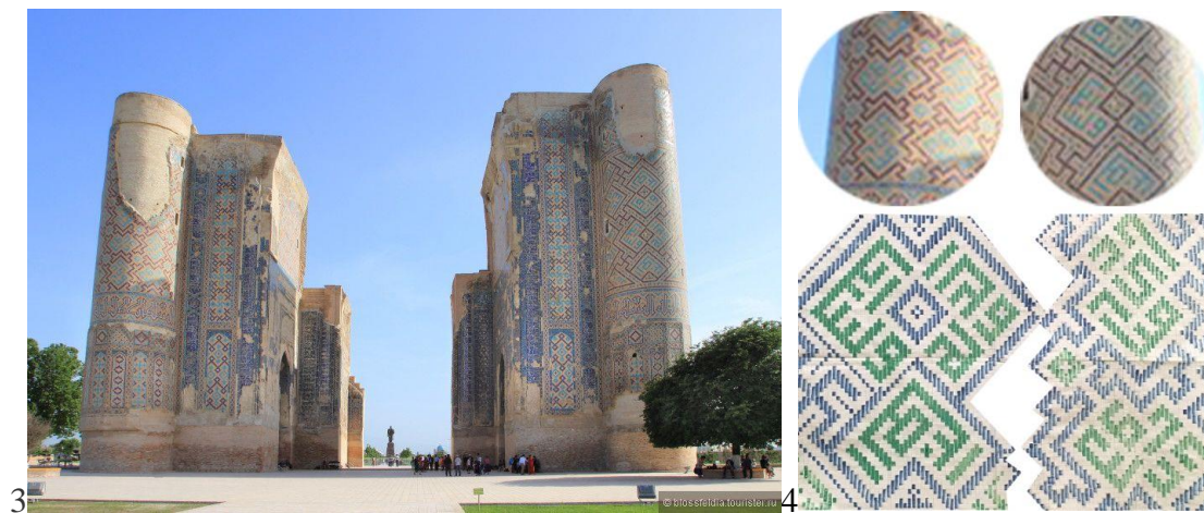
(Figure 3) The White Palace is a memorial in Shakhrisabz. Built by Amir Temur. (Figure 4) Words written on the tower floor on either side of the White House.
