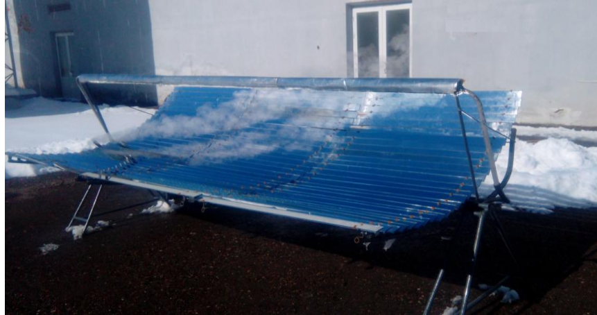
Fig. 4 b. Parabolic cylindrical solar plant based on linear mirrors
