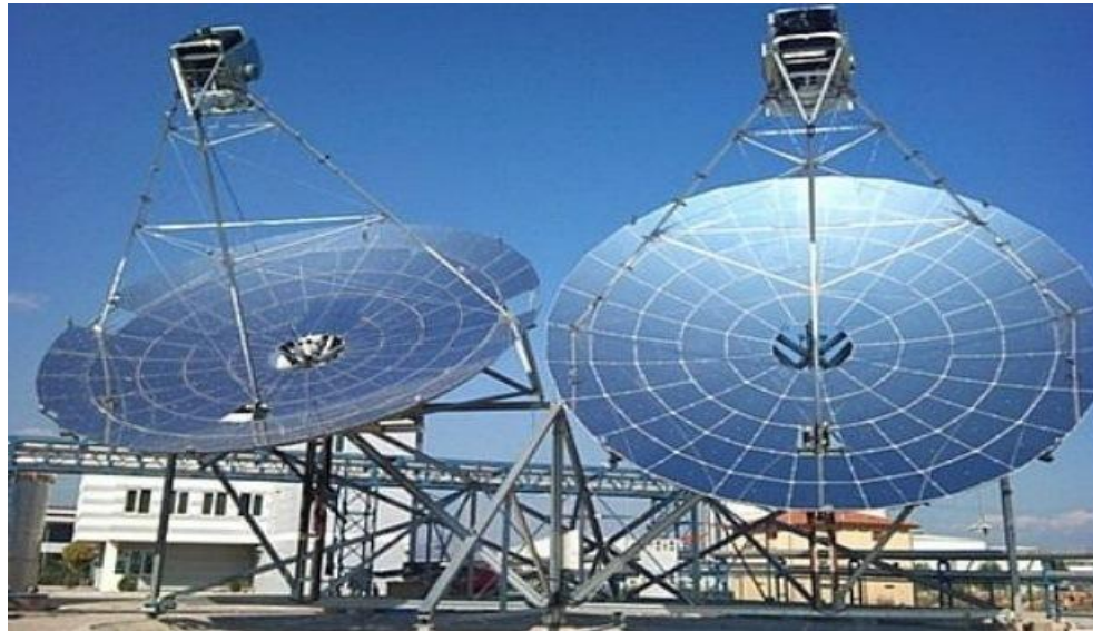
Fig. 6. Sector arrangement of the mirrors of the paraboloid concentrator [3]
