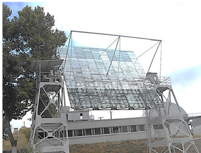
Fig. 5. General view of the Fresnel mirror - concentrating system (FMCS) on a flat base with dimensions of 10x10 m [10]
