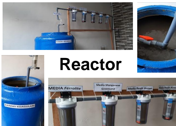
Fig. 2: Installation of Coagulation, Ferrolite, Manganese Greensand, and Resin
