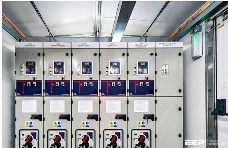
Figure 3 medium voltage switchgear [electrical-engineering-portal].
