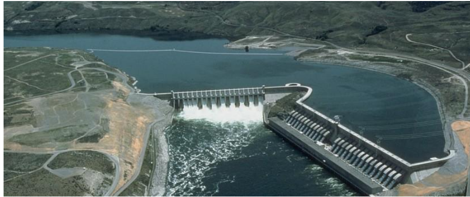
Figure1 Hydro-electric power plant
