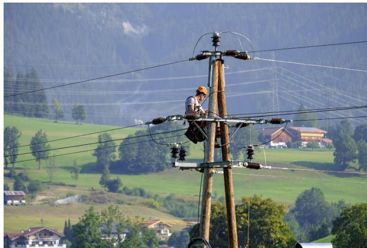
Figure 1 Transmission line maintenance.
