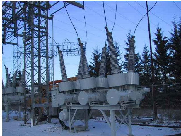
Figure 2 Sulphur Hexafluoride Circuit Breaker
